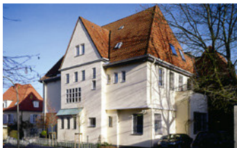
Head Office in Osnabrück
