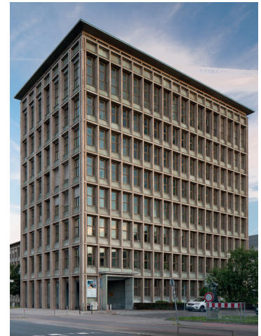
Former Preussag administration building in Hannover/Das ehemalige Preussag-Gebäude in Hannover
