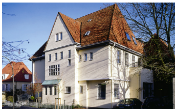
Head Office in Osnabrück
