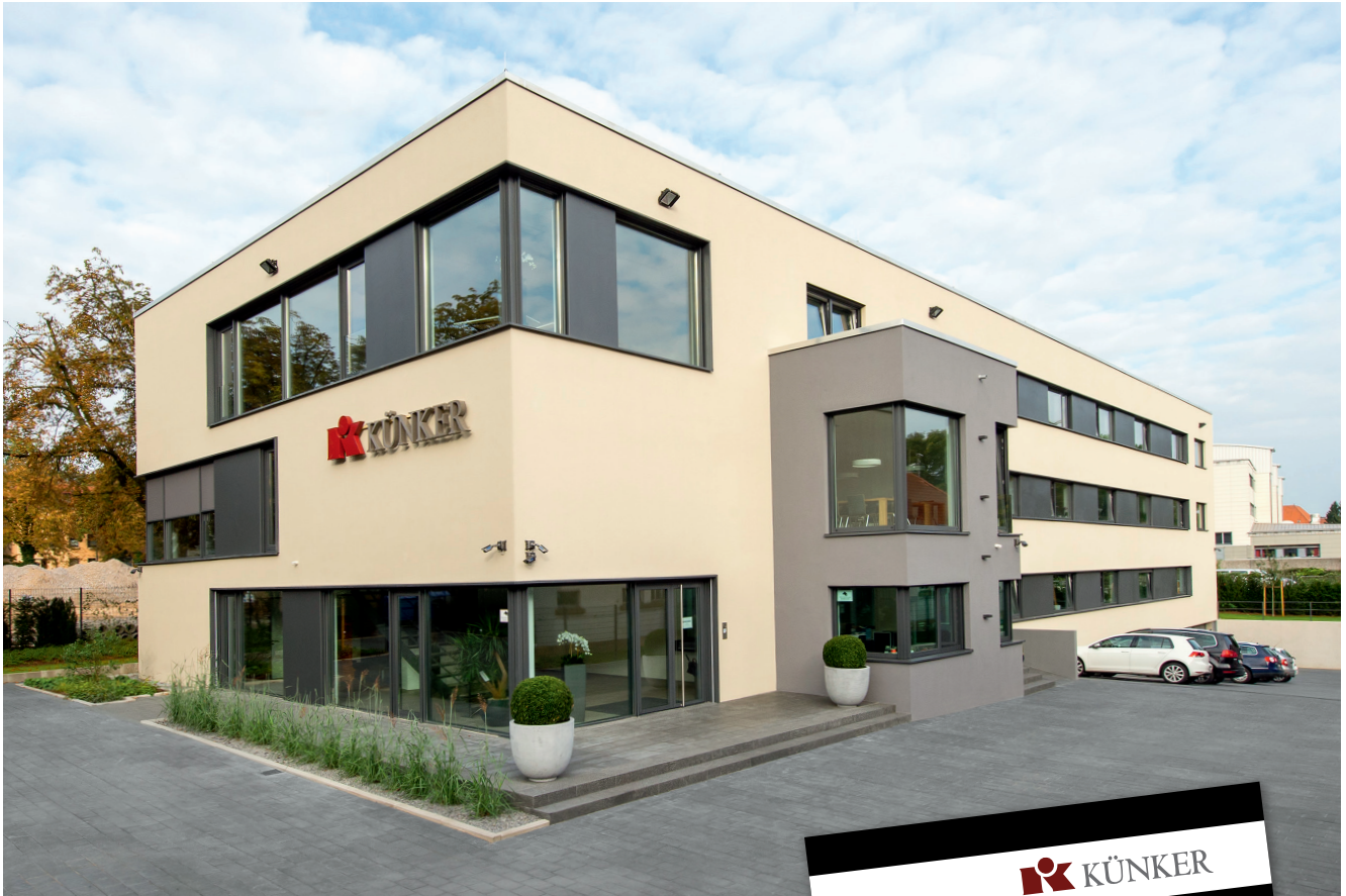
Der dritte Umzug 2014: Nobbenburger Straße 4a, Osnabrück The third company move in 2014: Nobbenburger Strasse 4a, Osnabrück
